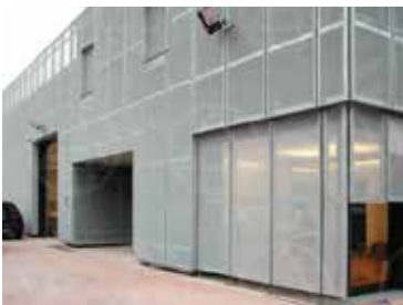
Manufacturing Warehouse Walls
